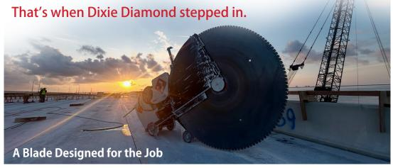
Working in collaboration with the customer's fabrication team in Grand Rapids, Michigan, Dixie Diamond engineered a fully customized 94" saw blade tailored specifically to the project's needs. Built to power through vertical diaphragm splits, pile cap sections, and heavily reinforced concrete, this blade delivered a level of performance that off-the-shelf options simply couldn't match.
